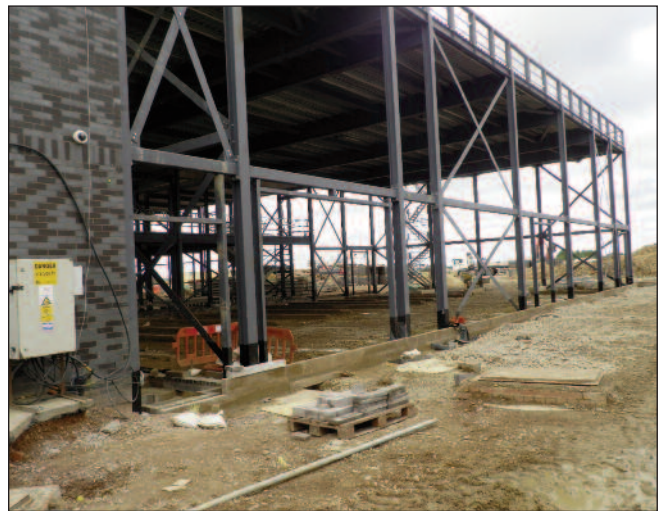
WINGING IN: The new 'orange wing' under construction.
