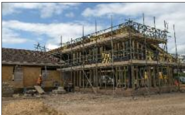
UNDER CONSTRUCTION: Work is progressing on Gamlingay Village Primary.
